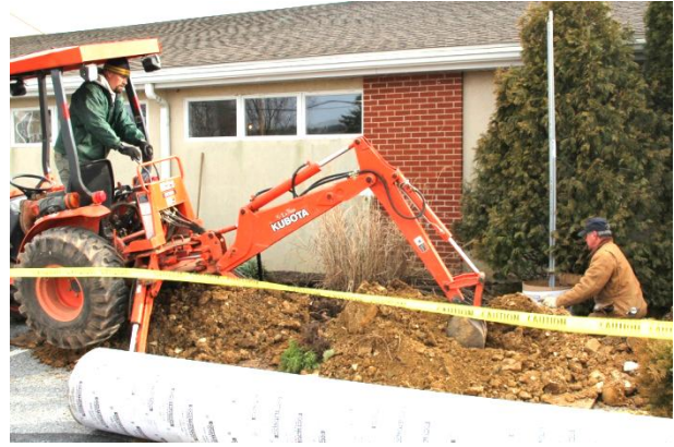
Matt Carter digs as Carl Stoltzfus prepares a mold for cement.
